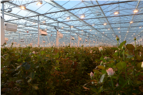
Figure : 4 ha commercial rose greenhouse
